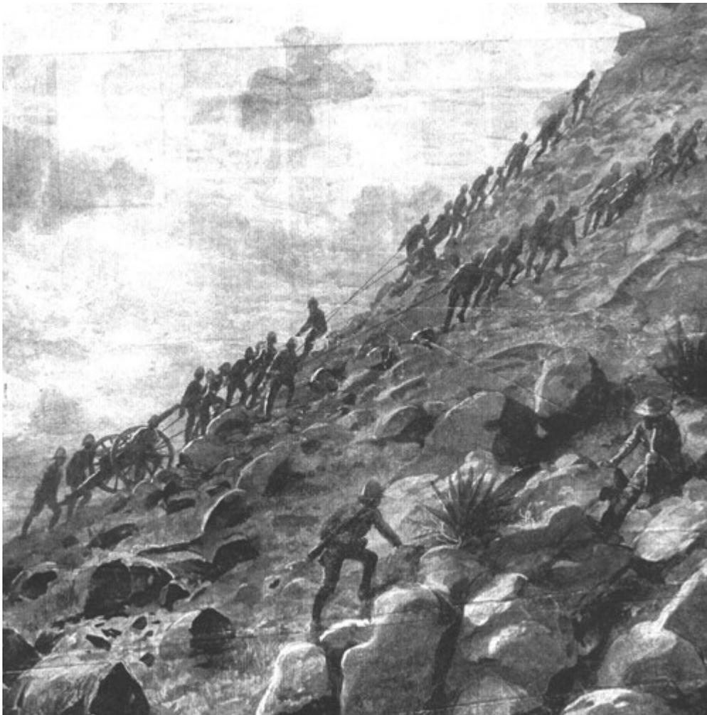
Because the loose stones and rocks made the hauling of food, water and ammunition an arduous task, an ammunition lift 1,400 feet long, made of 7 strand railway fencing wire was rigged up from the bottom to the top of **Coleskop**. 24ft rails were erected at the top and bottom as uprights. A second lift was made later by fixing a large drum between the two uprights on the top so that both lifts could be worked with the same hauling wire.
